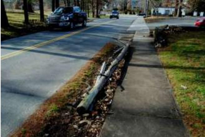
This is a serious road hazard created by the damaged utility pole projecting climbing spikes, tubes and wires to snag a pedestrian or a vehicle swerving to avoid oncoming traffic on Tabor Street right in front of Tabor Church.
